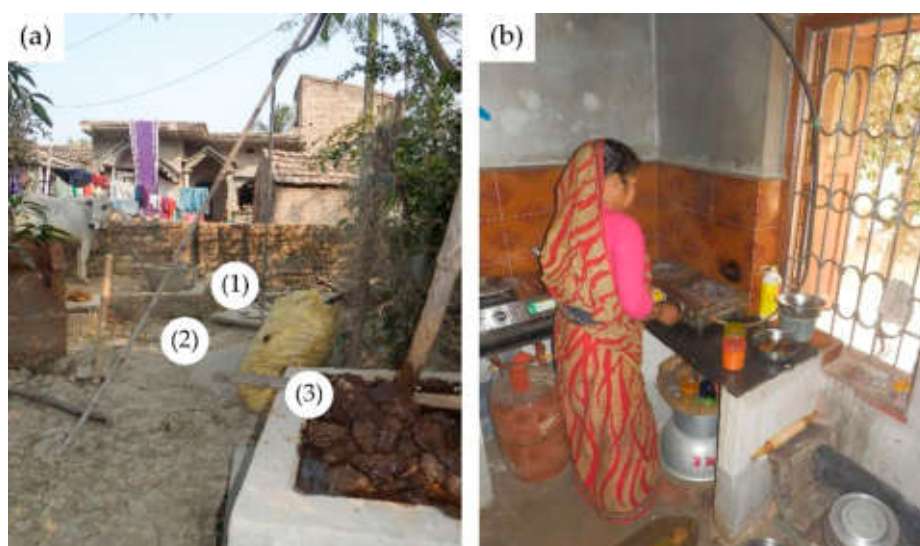
Figure 7. Household biodigester (a) Deenbandhu Model: (1) inlet filled with manure and water; (2) underground fixed-dome fermenter, and (3) outlet chamber in the rural village of Ghoragachha, West Bengal India. (b). Women cooking on a biogas stove, directly connected with the biodigester.
